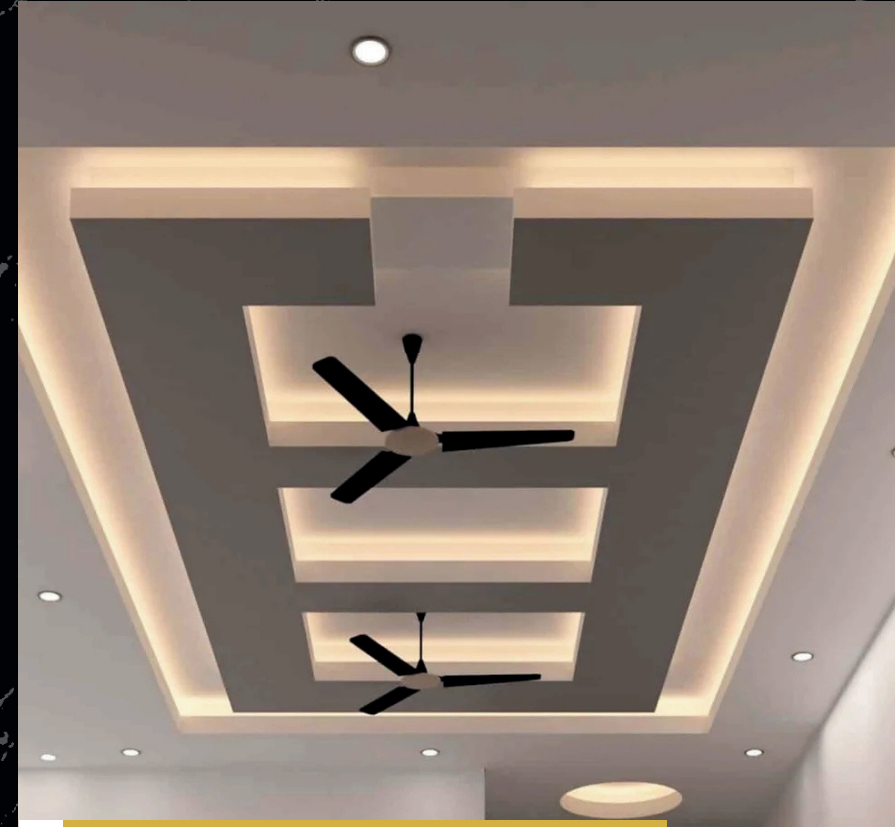
FALSE CEILING WITH CONCEALED LIGHTING
